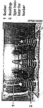
Busbar compartment extending over 3 panels (example 17.5 kV) Side view
